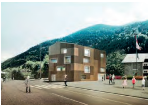
CENTRE DU VILLAGE | BFIK (2013_Troistorrents)
