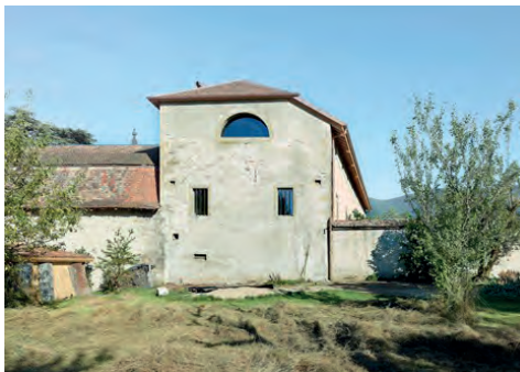
TRANSFORMER GRANGE | PICTET CHARLES (2012_Landecy)
